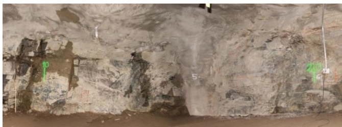
Figure 4. Photo of the 10-20 tunnel section.
