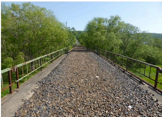
Fig. 5. Evenly distributed ballasts on the bridge.
