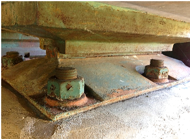
Fig. 4. Line-bearing support.
