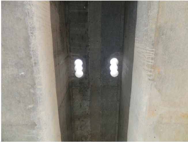
Fig. 7. Holes on the slab for lifting.
