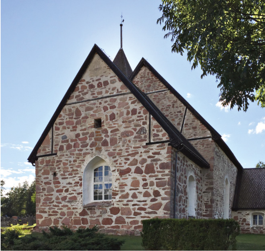
FIGURE 7 Hammarland church with both tie beam truss and rafter foot truss visible in the gables
