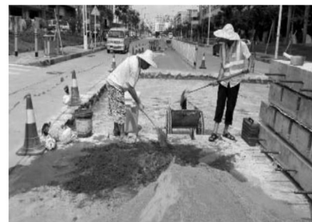
Fig. 57. Prefabricated pavement base layer. (a) Sand cushion course (Tayabji, 2016). (b) Dry-mixed mortar (Tang, 2019).
