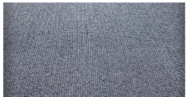
Fig. 76. Pavement texture after fine milling.
