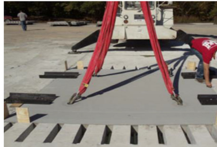
Fig. 54. Typical applications of the Michigan slab system. (a) Repairing road. (b) Repairing airport pavement.
