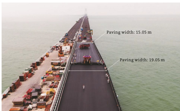
Fig. 71. Continuous widening paving of Hong Kong–Zhuhai–Macao Bridge.
