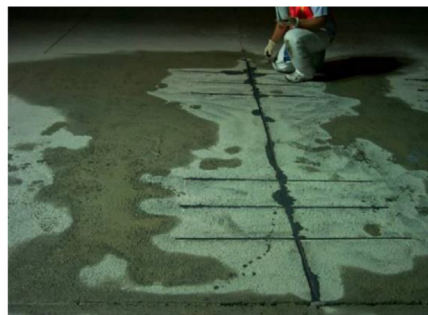
Fig. 55. Typical application of Uretex stitch slab system. (a) Repairing the pavement. (b) Reinforcing the road.
