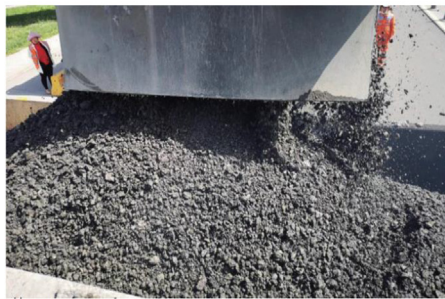
Fig. 78. Construction site of W380CR foam asphalt cold in-situ recycling unit. (a) Homogeneous foamed bitumen cold recycling mixture. (b) Intelligent and efficient regeneration.
