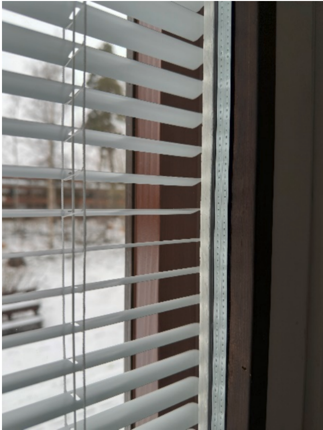
Fig. 3. Example of window with blinds between panes.
