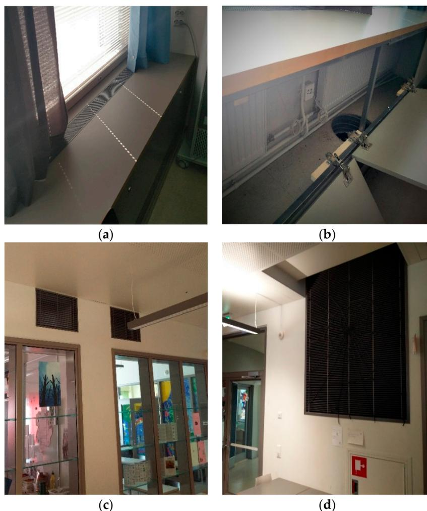
**Figure 3.** (a,b) Supply air grill and duct in the classrooms; (c) transfer air grilles in the partitions between classrooms and the lobby and (d) exhaust stack in the lobby.
