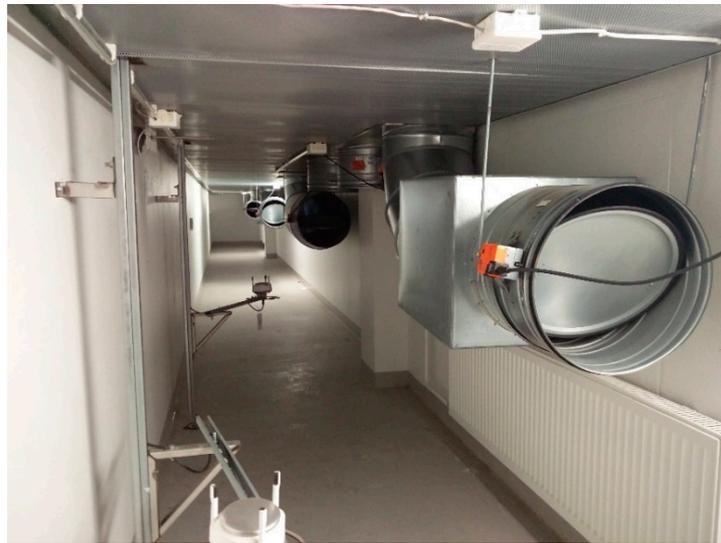
**Figure 4.** Supply air duct corridor and classroom-specific ducts' terminal units in the basement. Dampers are opened 20%, as designed.
