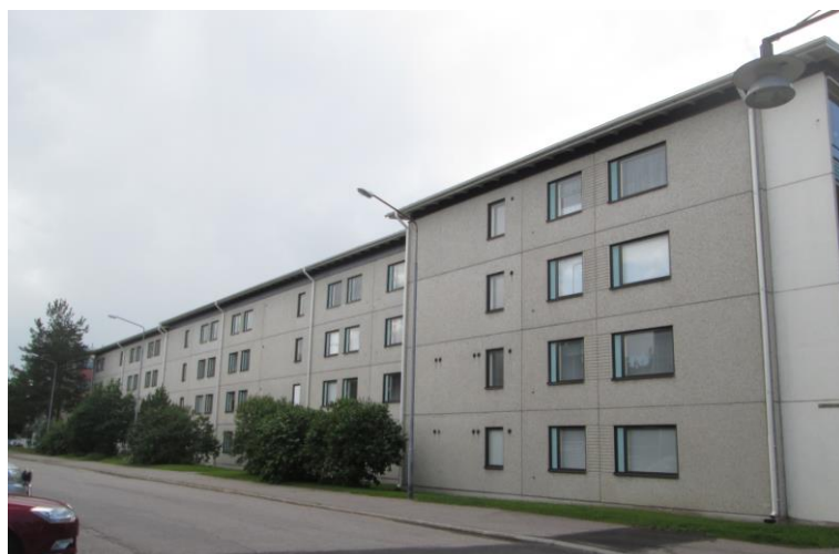
Figures 2-4. Cases illustrated. To demonstrate the suggested evaluation method three options of building envelope retrofits are assessed. The images illustrate built examples. From the top; A) a building envelope retrofitted using prefabricated timber-based element systems ( TES EnergyFacade ), B) a retrofit using thermal insulation and rendering (conventional) with new windows and glazed balconies, and (C), a facade with upkeep consisting of continuous maintenance and optional glazing of balconies. All buildings originate from the 1970's, were built using similar building plans and the same structural concrete system. Images by the author.
