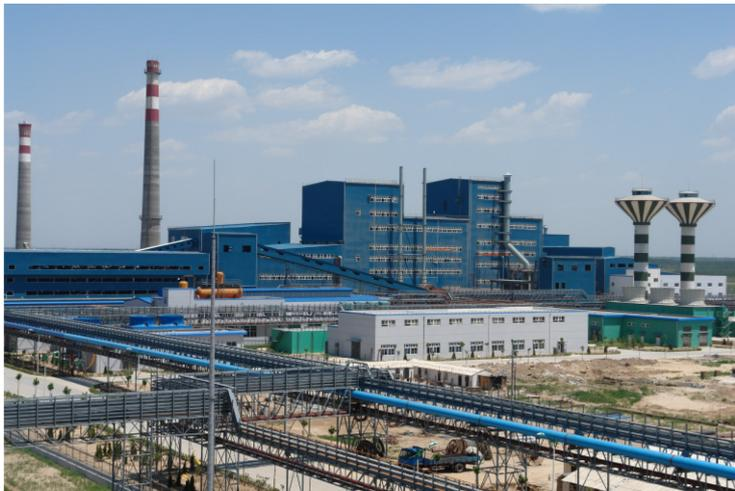
Shandong Yanggu Xiangguang Copper Co. Ltd was the second copper smelter in the world to adopt the FCF technology, Fig. 14. Its production started in September 29, 2007. One of the main reasons for the decision favoring Outotec FSF and FCF processes for the green field smelter in China are increasing environmental concerns. With the FCF process, sustainable operation offers the smelter an environmental license to operate for decades to come.
