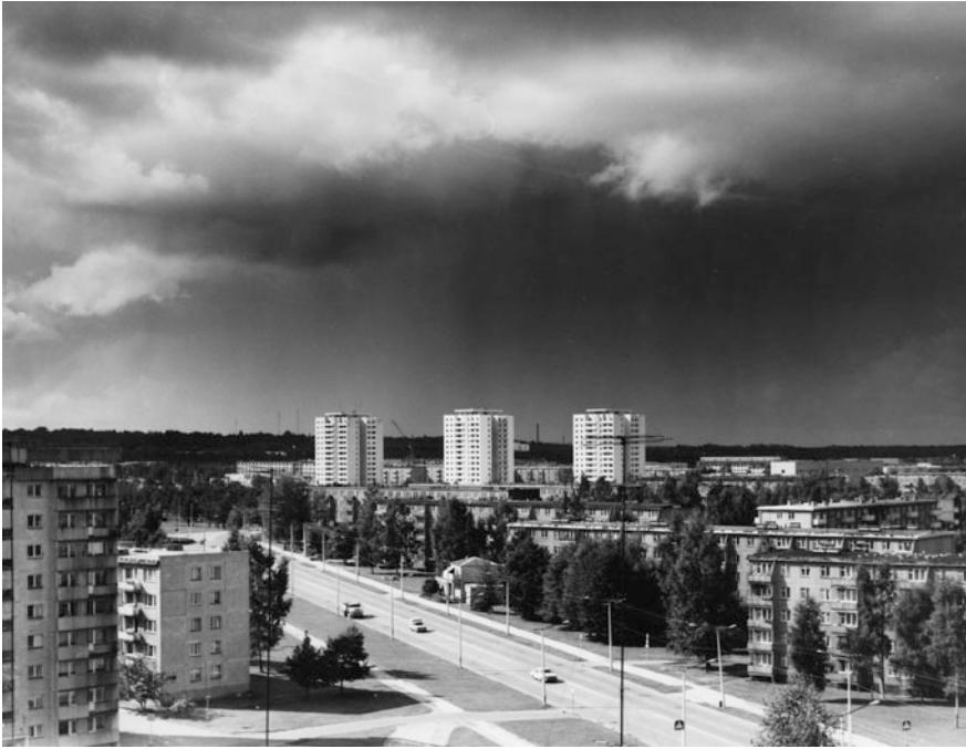
Fig. 5.5 The first mikrorayons of Mustamäe estate in Tallinn (1958–73) consist of 4- to 5-floor apartment blocks built with 1-464 standard. Source Museum of Estonian Architecture, used with permission
