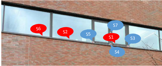
(b) Arrangement of the seven Sensortags on the building facade.
