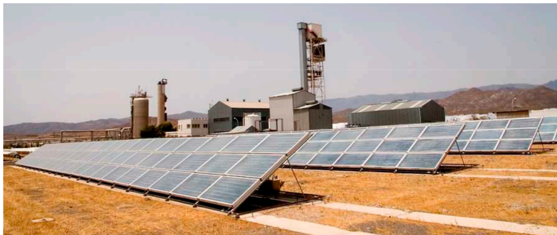
Figure 40. A 500 m 2 stationary CPC solar collector field [74].
