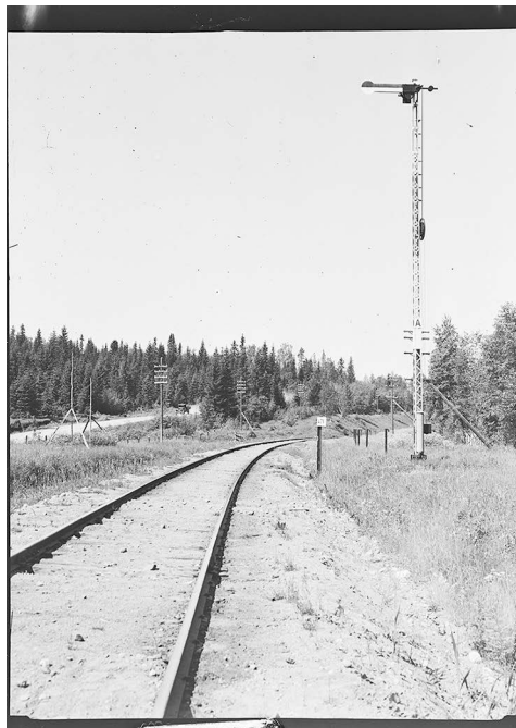
Figure 11: A semaphore main signal preceding the Kallavesi swing bridge from the south by Gustav Rafael Roos
