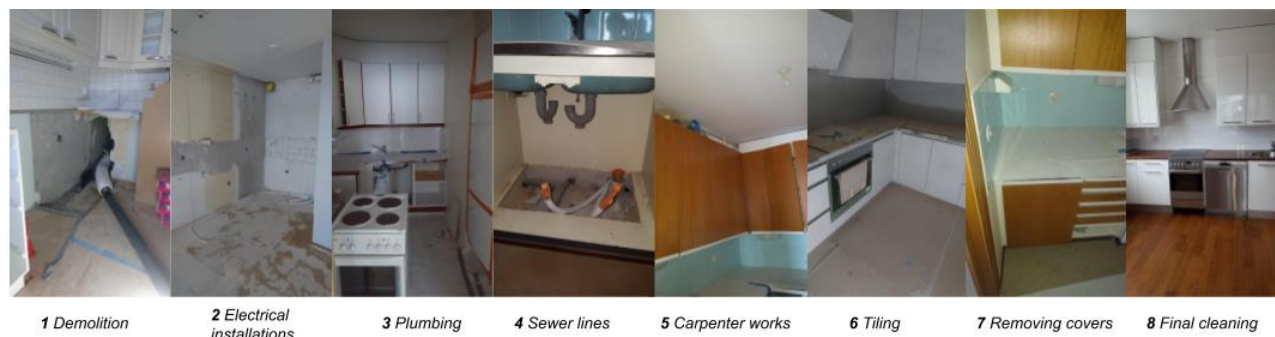
Fig.4. Example photos of 8 stages of kitchen innovation.
