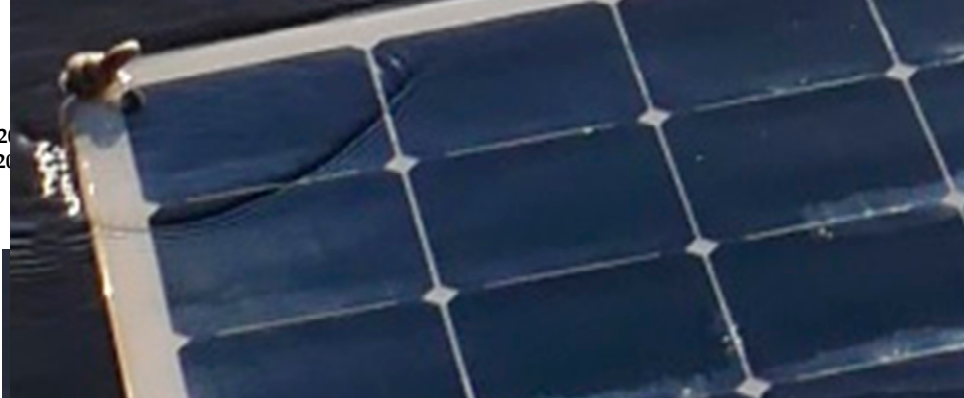
Figure 2. Closeup of floating photovoltaic/floatovoltaic (FPV) corner after deployment, showing water coverage from a modest wave (top left).
