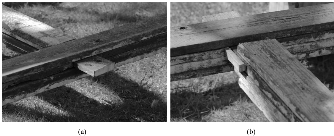
Figure 10: Joining details: (a) slide-in joints, and (b) inserted wedge made from salvaged plywood.
