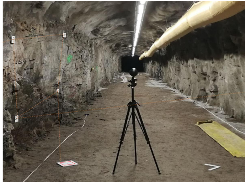
Figure 1. Photo depicting part of the tunnel section that was selected for testing the 360-degree camera for photogrammetric digitization and remote rock mass mapping. Control distances were measured between the control points mounted on the tunnel wall (example illustrated with an orange dashed line). An orientation board with four control points was placed on the floor (white board in the lower left corner) and was used to orient the model.
